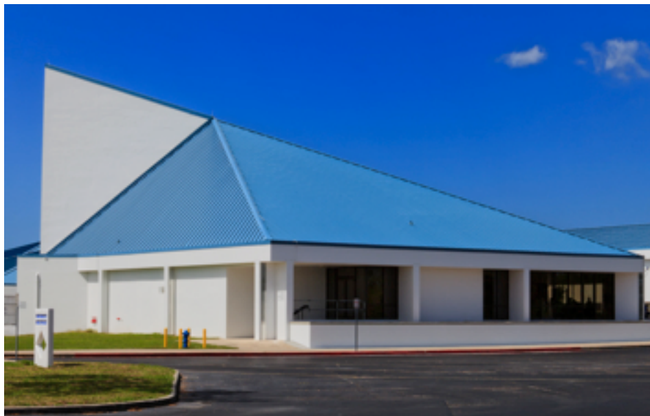
East Lake High School - Tarpon Springs, FL - Architect: C.B. Goldsmith Winner of 2013 of FRSA STAR Award for Roofing Excellence.
